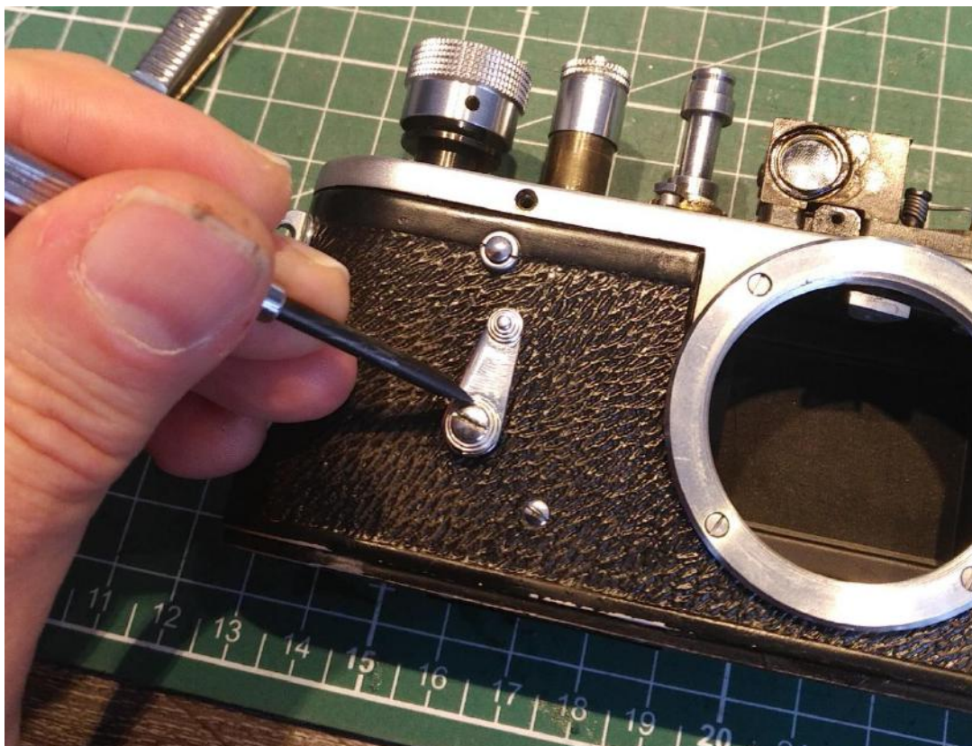
Removing the self-timer lever.
